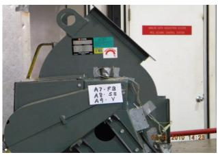
Floor mounted - isolated using (4) Caldyne Model JQA-V-E143 with unit mounted to 3/8" stud on top of isolators and each isolator was welded directly to the table.
