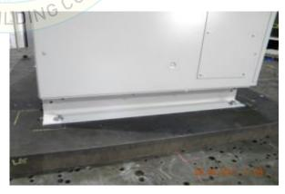
Base mounted - rigid with (4) 1/2" - 13 Grade 5 hex-head bolts, washers, and lock washers.
