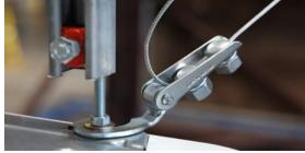
The UUT was ceiling hung using four (4) A36 hanger rods w/rod stiffeners and four (4) 1/8" cable braces w/ Mason SCB-1/SCBH-1 clips at each end.
