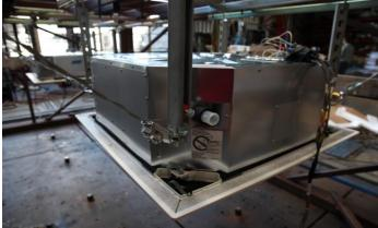
The UUT was ceiling suspended using four (4) 3/8" A36 hanger rods w/rod stiffeners & four (4) 1/8" cable braces w/Mason SCB-1/SCBH-1 clips at each end. Future installations will require (8) perpendicular cable braces minimum to restrain against torsion.
