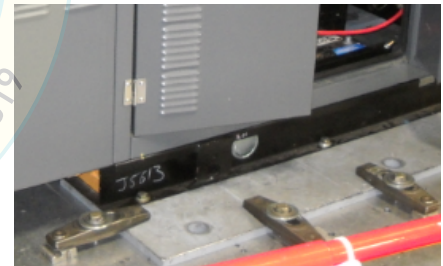
Figure 3.2: Mounting Detail
