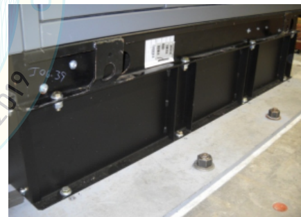
Figure 2C.2: Mounting Detail
