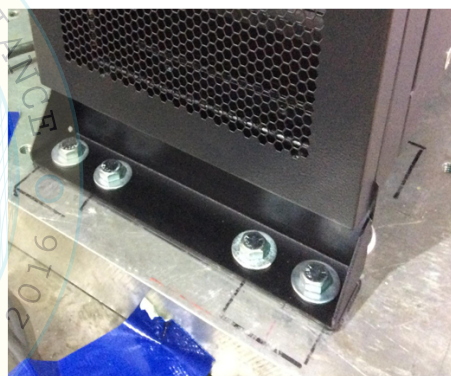
Figure 5C.2: Mounting Details with Modifications
