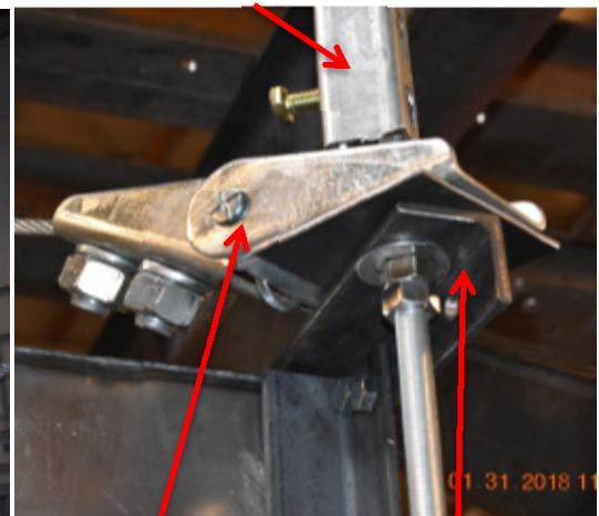
Mason SCBH-2 2" x 1/4" Steel Angle
