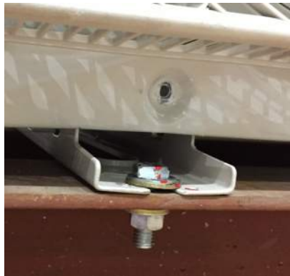
Figure UUT-3.3: Lower left front screw fell out during test- base material pullout failure
