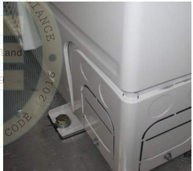
Figure UUT-D2.2: Mounting Details
