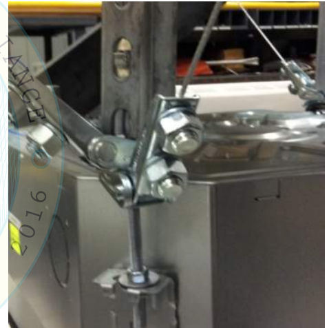
Figure UUT-G2.2: Detail of brace connection
