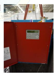
Unit mounted to wall fixture with five (5) 1/4"x 3/4" wood screws. Washers were used in additon to the wood screw at each corner.
